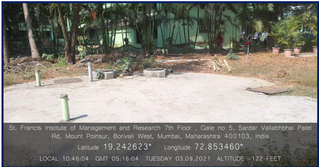
Water gets stored in underground Circular Well
