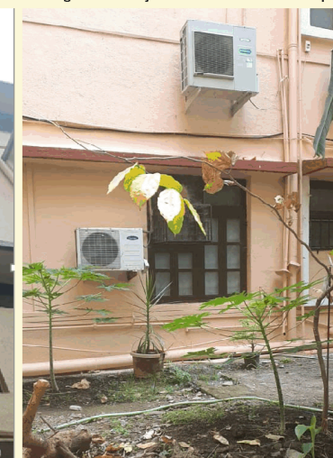
Brought Down by Vertical & Horizontal Pipes
